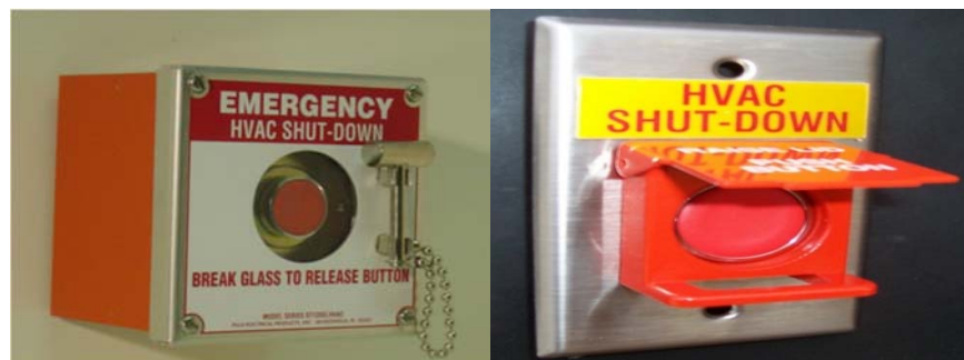
Figure 7. HVAC Shut Off Switch
