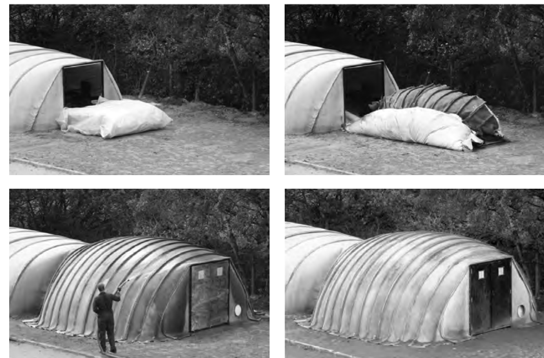
Figure 4: Detailed traditional deployment of Concrete Canvas. (Top Left) Delivery. (Top Right) Inflation. (Bottom Left) Hydration. (Bottom Right) Setting. - photos courtesy Concrete Canvas
