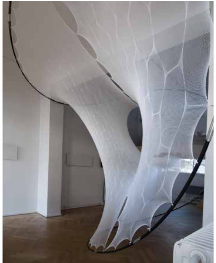
Figure 10: Semi-Toroidal Textile Hybrid installation at ggggallery in Copenhagen, Denmark, composed of GFRP bending-active boundary and two tensioned textile elements (Sean Ahlquist, Institute for Computational Design—Professor Achim Menges, University of Stuttgart 2012)
