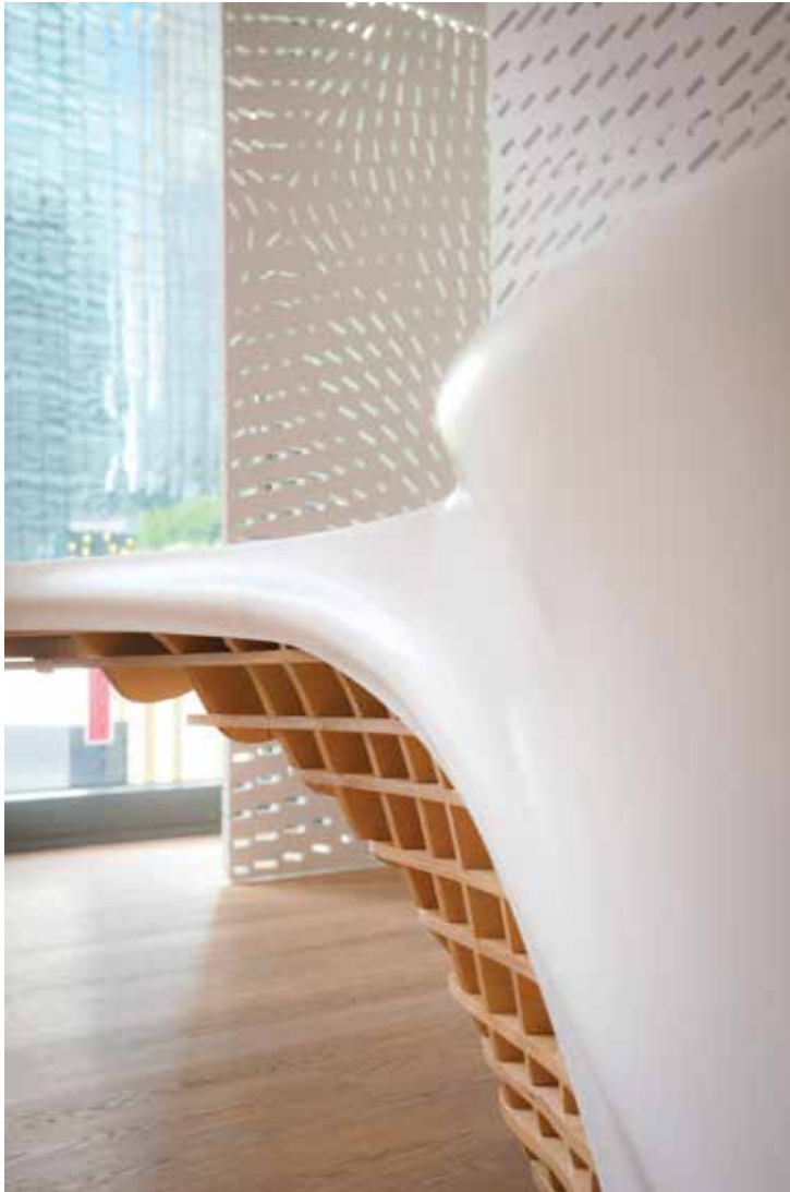
Figure 10: Final detail with egg-crate and compound curvature of the shell.
