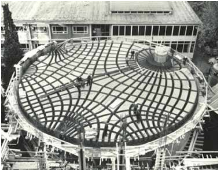
Figure 3: Formwork represented 80% of the construction costs for the slab of the Zoology Lecture Hall of the University of Freiburg, designed by Hans Dieter Hecker in 1969 (Antony et al. 2014).
