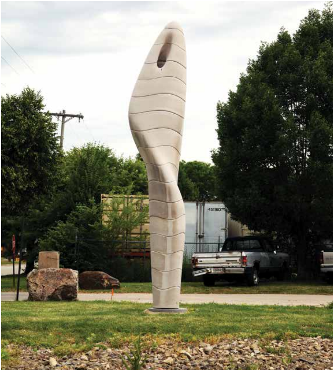
Figure 17: Full-scale prototype consisting of 17 unique dry-stacked drums on site.
