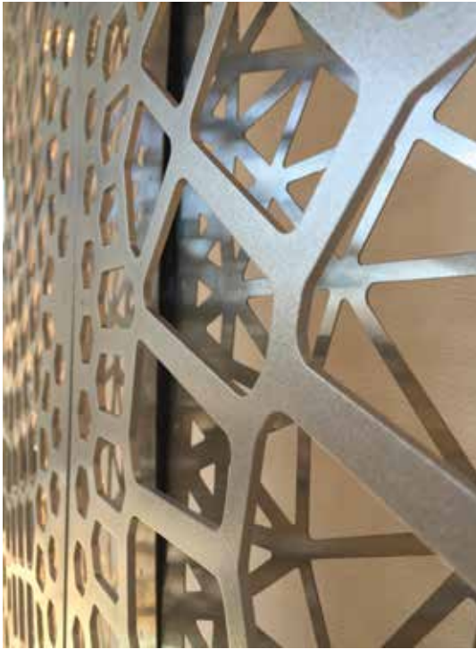
Figure 10: Detail views of CNC-milled and powder-coated exterior skin vs. laser-cut and PVD-coated inner skin.
